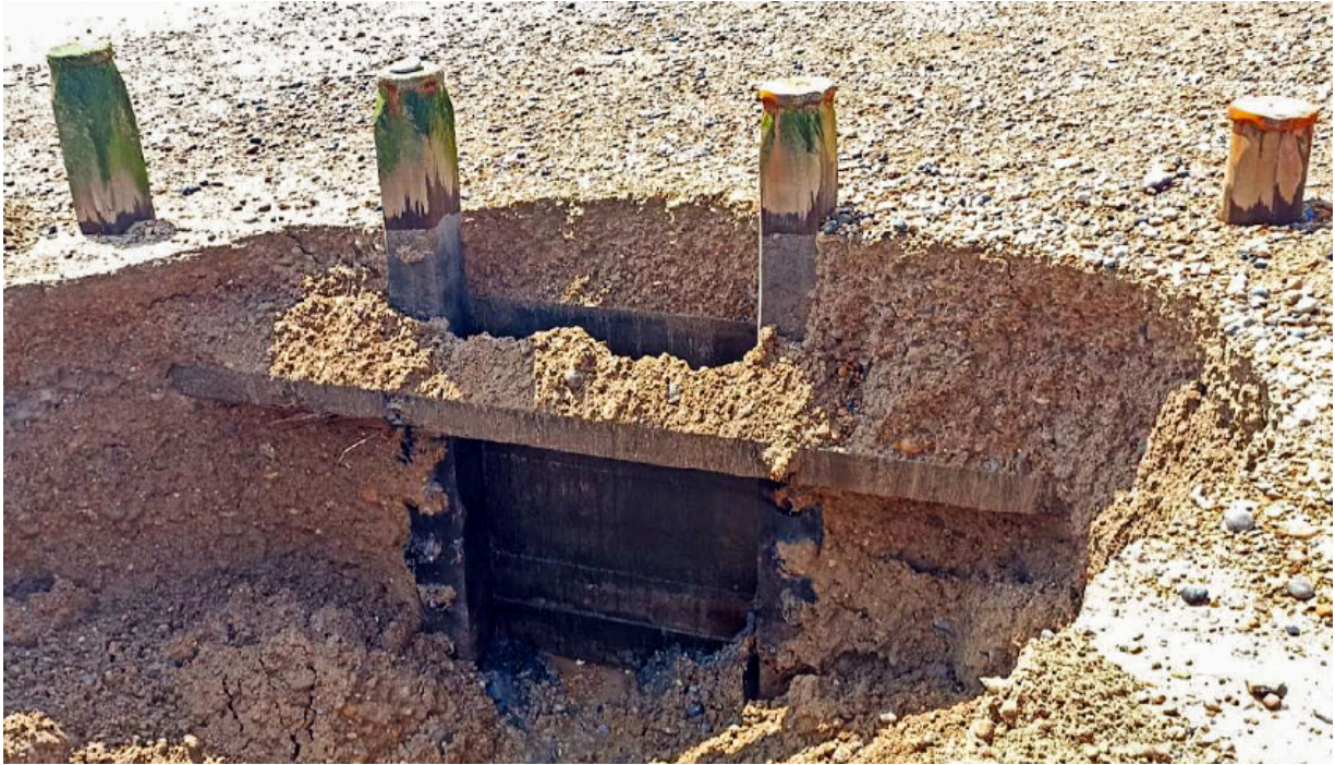
Photo: Beneath the surface of a groyne showing it to be in good condition
