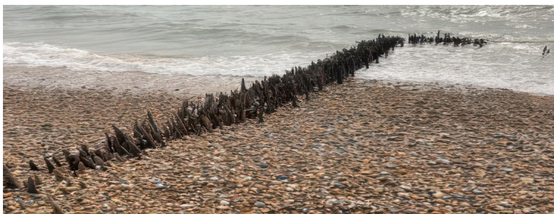
Photo: Timber fascines in the shingle
