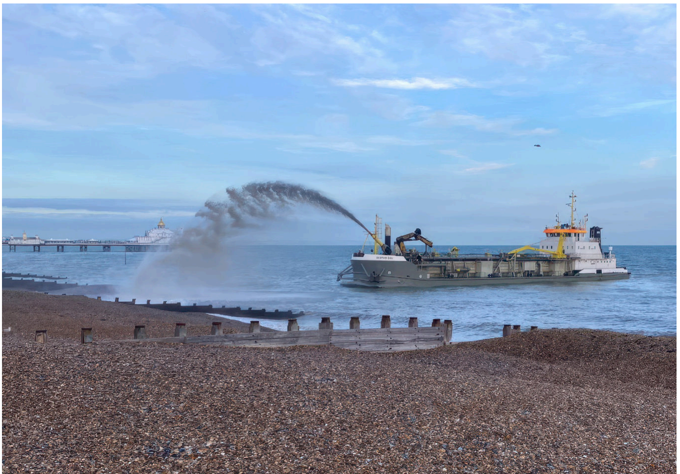
Photo: Dredger Sospan Dau pumping shingle onto Eastbourne beach
