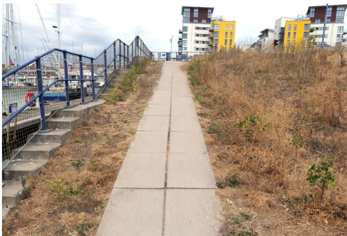
This paved slope is now the only access up and down. It needs hand rails.
