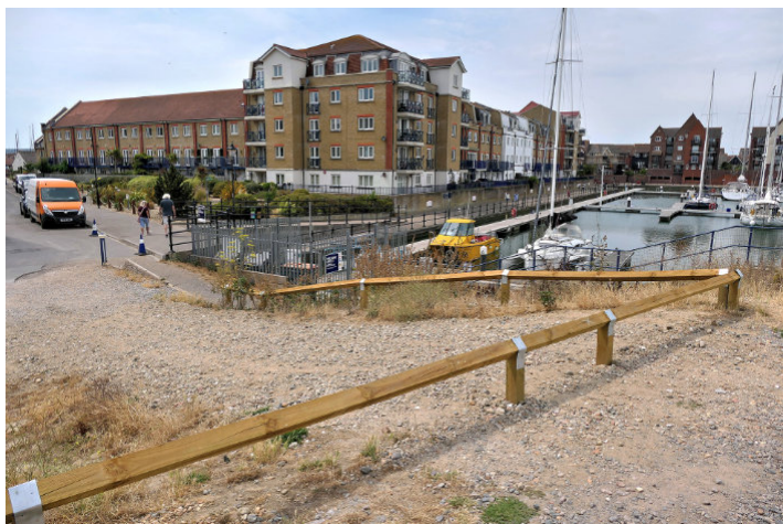
The other fenced off slope
