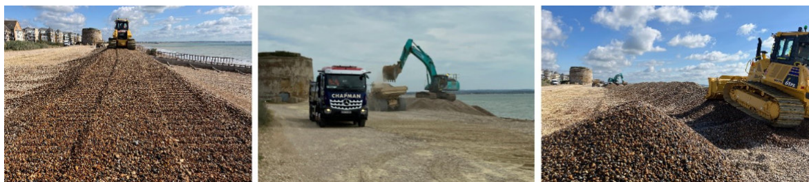
Photo: Beach replenishment works using recycled shingle from the Hastings trial
