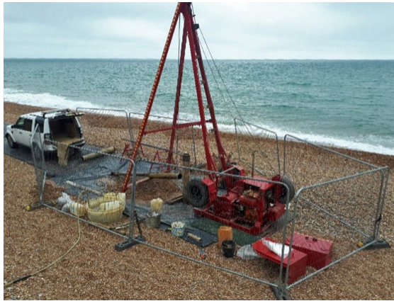
Photo: Typical set-up for ground investigations, including drilling equipment and temporary safety fencing
