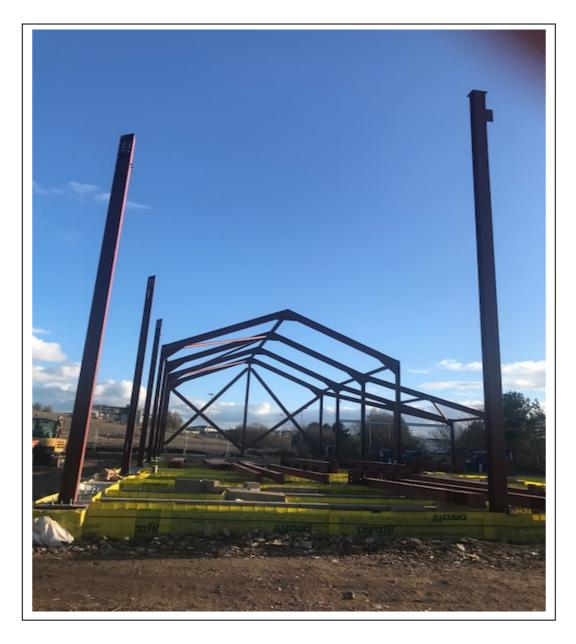
Steelworks are expected to complete early next week. Floor beams will progress from the start Of the week. Brickwork will commence once the floor beams are in situ, likely the end of the Week. Steelwork was affected by high winds.
